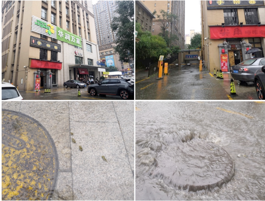
Figure 1. Combined sewer overflows from manholes during an urban flooding event in China (Han and He, 2021)
